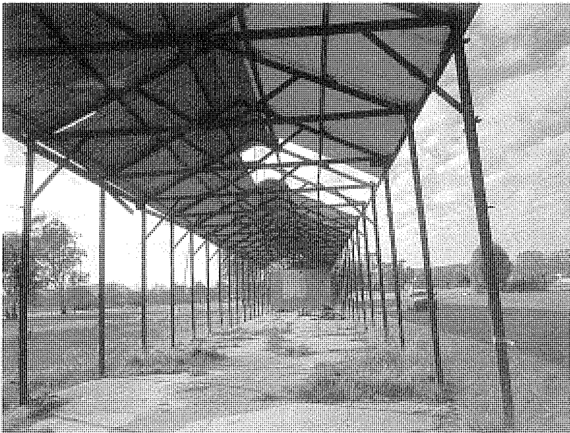
Internal Roof – Looking East
