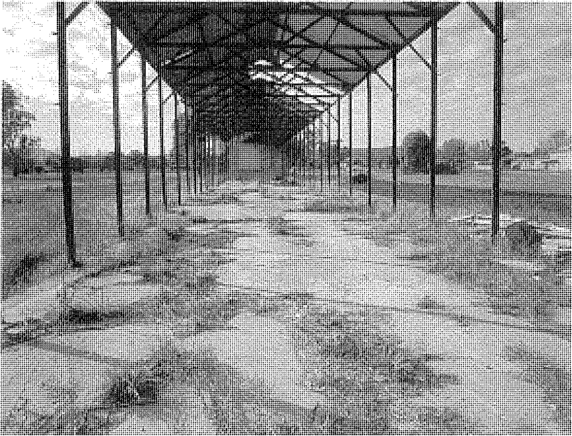
Internal – looking East
