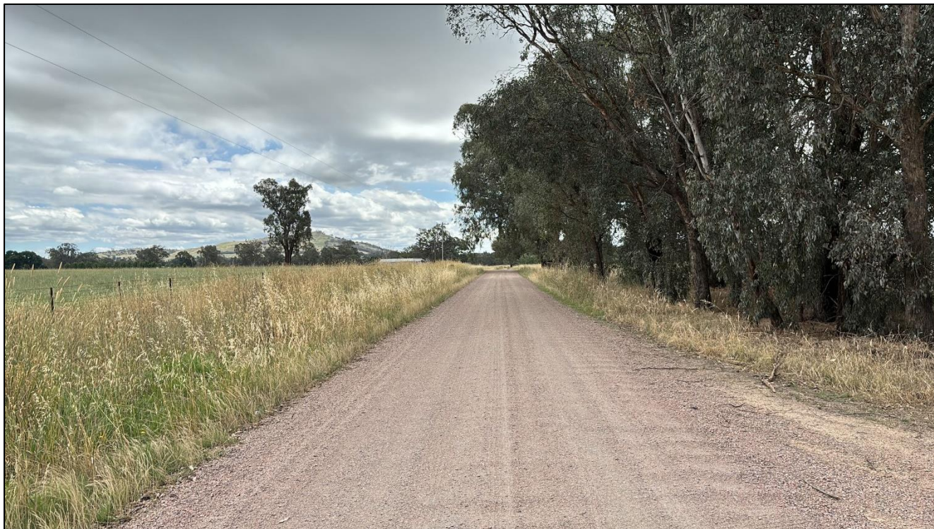
Figure 5: Bendemeer Lane, looking west at the subject site driveway
