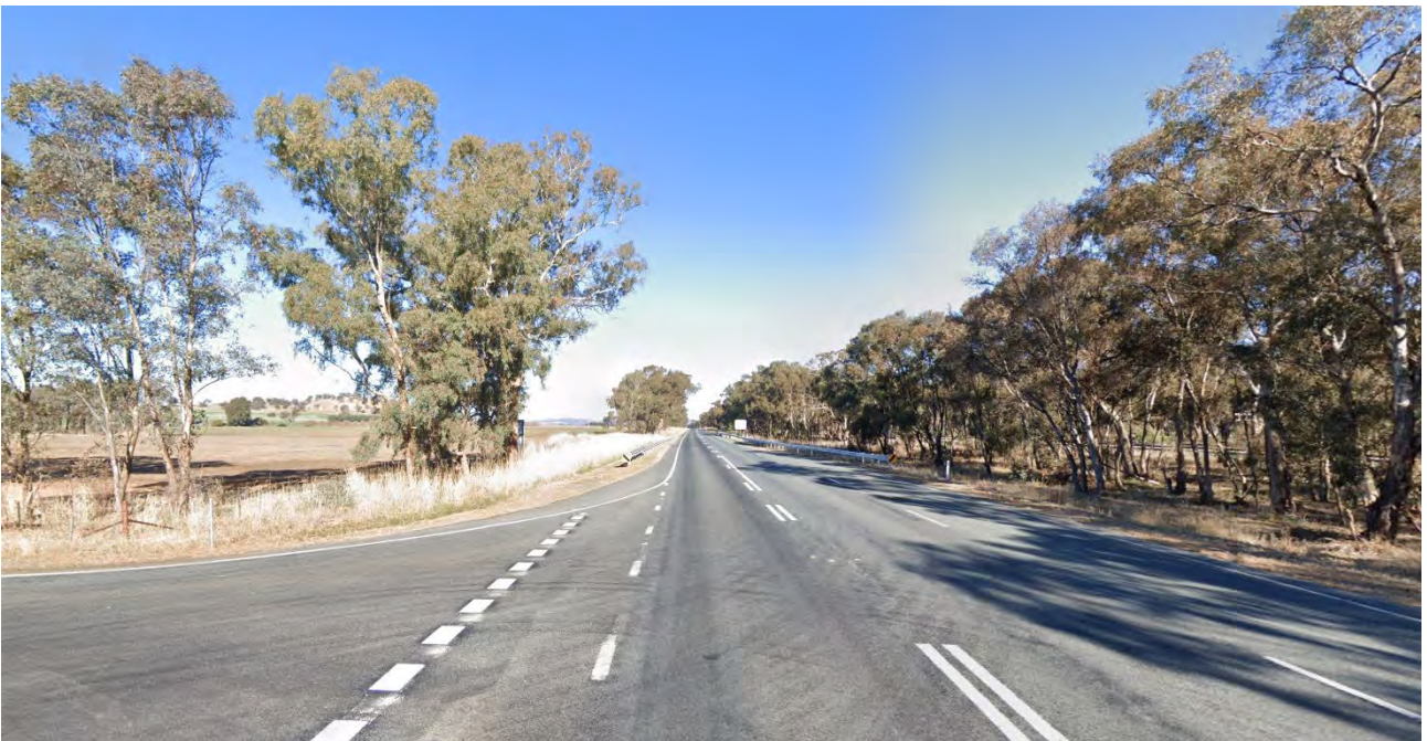
Figure 10 Olympic Highway looking South showing AUR
