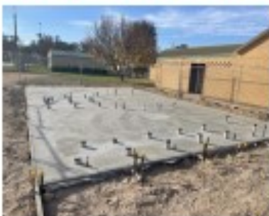
Stage 1. The New Toilet.
