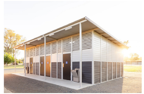
Pic Burrumbuttock - New toilet facilities. Photo courtesy of Modus
