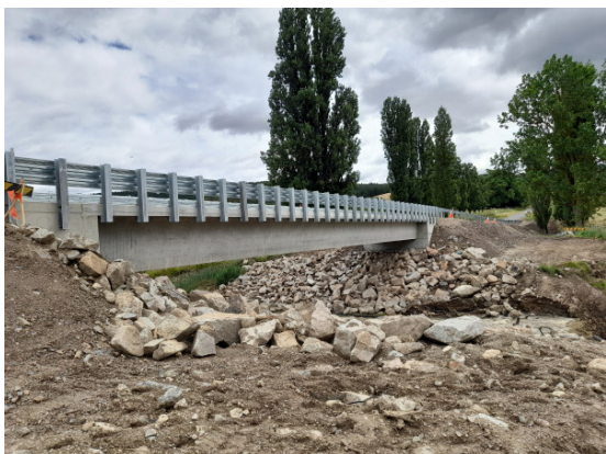
Pic Coppabella Bridge along Coppabella Road
