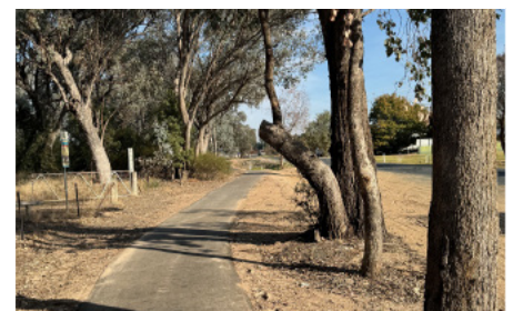
Pic Culcairn - The completed Bike Path upgrade.
