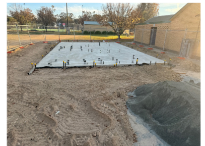
Pic Burrumbuttock - Concrete slab poured for the toilet building.
