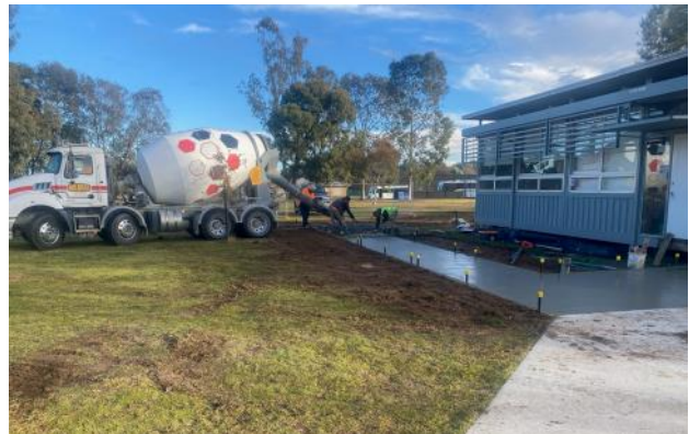
Progress to paths and wheelchair access
